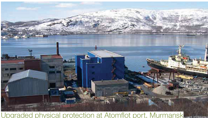
Upgraded physical protection at Atomflot port, Murmansk
