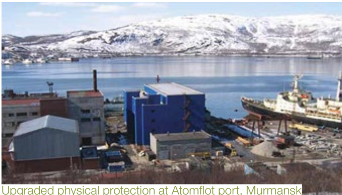
Upgraded physical protection at Atomflot port, Murmansk
