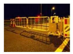
A new system to protect highways teams at work access points has been successfully launched. Devised by Colas and development partners Solar and Electric Gates Ltd (S&EG), the new Readi-Guard system opens access gates to work areas remotely removing the need for manual operation.
