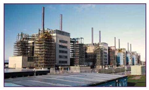
Since the project began eight years ago. 3.300 tonnes of asbestos have been removed from the turbine hall, four reactor buildings and 16 heat exchangers. More than one million bags of asbestos waste (equivalent to filling four Olympic-sized swimming pools) were despatched to licensed landfill sites.
