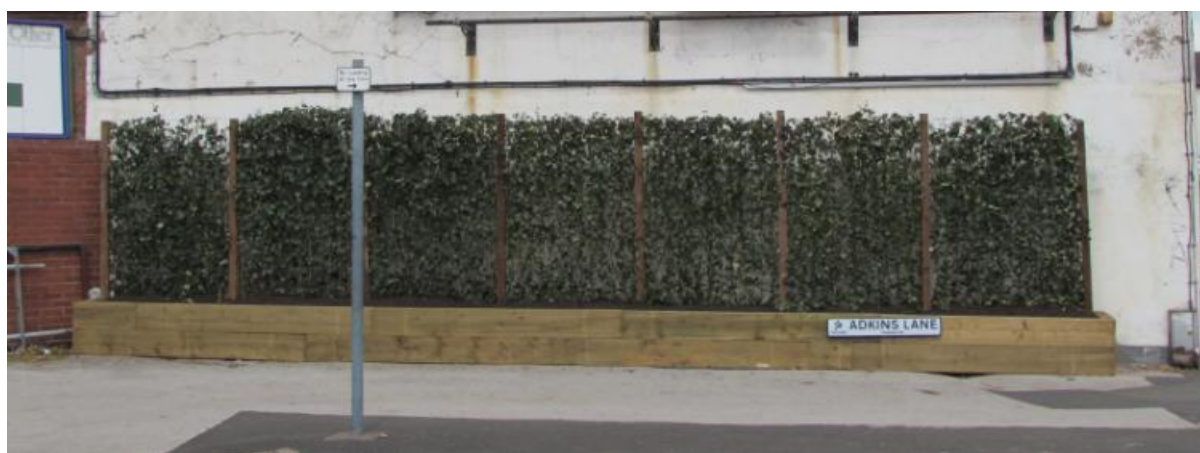
Figure 3: Green wall installation at junction of Adkins Lane and Bearwood Road © Sandwell Metropolitan Borough Council 2015
