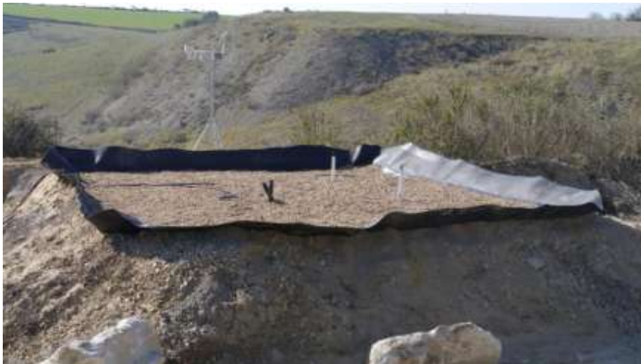
Figure 1 Completed test pad
