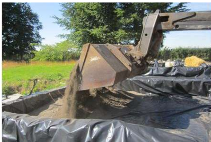
Figure 2. Construction of the PLA storage heaps
