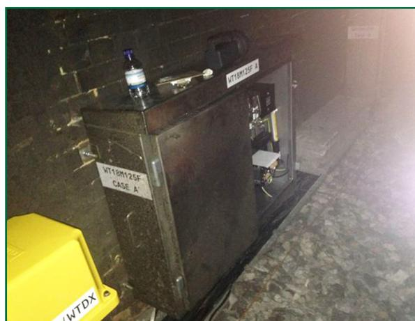
Figure 4: The cabinet as found after the accident with the right door missing
