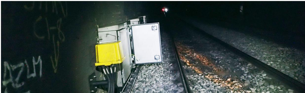
Figure 6: View from the cess adjacent to the up fast line looking towards London showing a reconstruction of the appearance of the door of Cabinet A fully open
