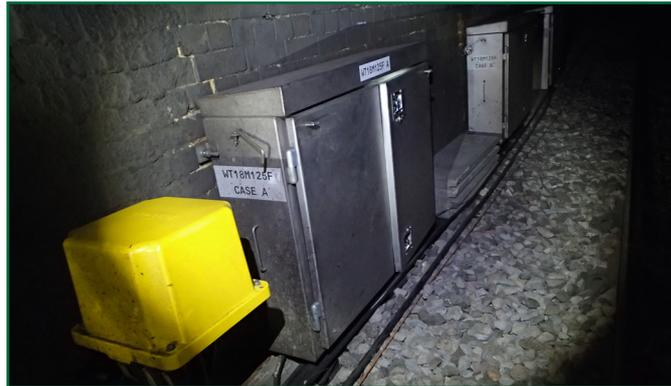
*Figure 14: View from the cess adjacent to the up fast line looking towards London showing a reconstruction of the appearance of the right-hand door of Cabinet 'A' slightly proud of the left-hand door*
