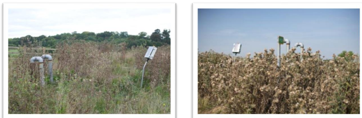
Figure 5-16 – Unmaintained planting plots potentially affecting access to drainage/ water attenuation equipment and PCDs
