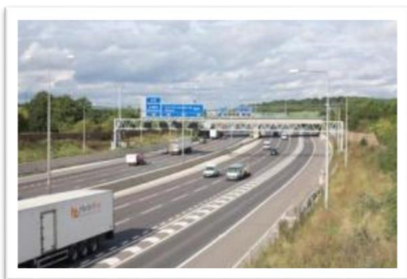
Figure 5-2 – Noise barriers that have been replaced at Nags Head Lane
