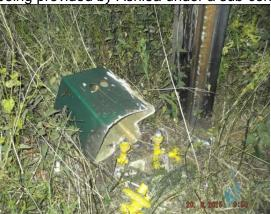
Whilst a 4X4 mower was cutting around a street name sign it made contact with a green box that was not visible in the long vegetation. The box covered a National Grid gas regulator between a medium pressure & low pressure service main. The contact caused damage to the apparatus resulted in a gas leak. A National Grid Gas Engineer arrived on site diagnosed the problem then
