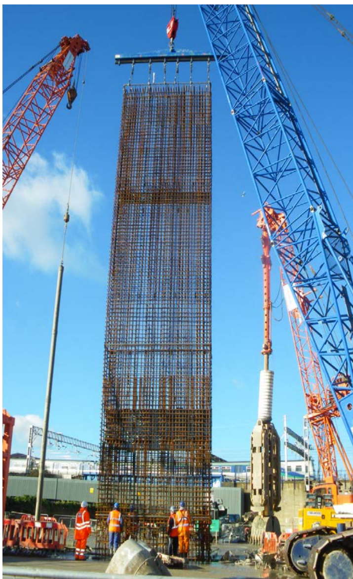
Figure 1: Installation of reinforcement cage for Crossrail diaphragm wall (for a deep shaft) with fibre optic sensors attached
