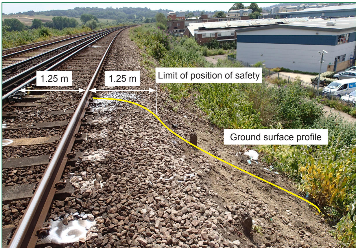
Figure 3: Location of accident, showing ground profile
