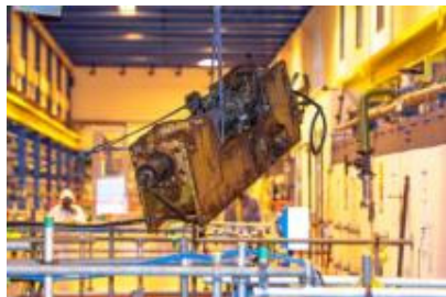
Material being removed from the Pile Fuel Storage Pond
