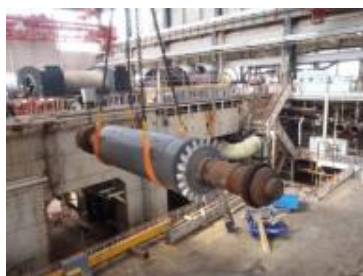
Dungeness turbine hall deplanting ready for demolition
