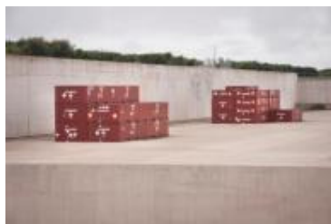
Vault 9 at the LLWR
