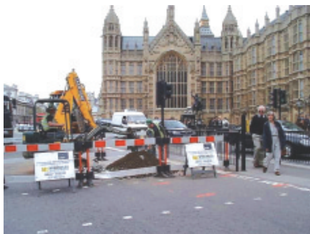
Pedestrians negotiating street works (Source: THUS Telecommunications)
