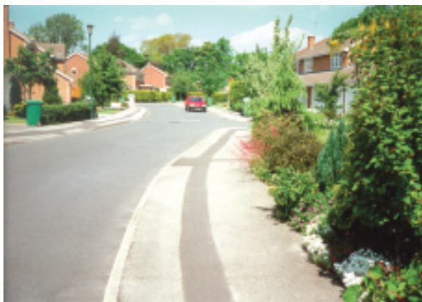
A telecommunications installation completed to a high standard of quality in compliance with the requirements of the NRSWA (Source: TRL Limited)
