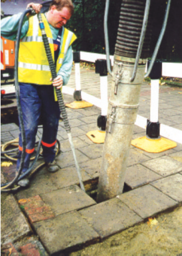
Excavation carried out by 'keyhole' surgery (Source: Transco)
