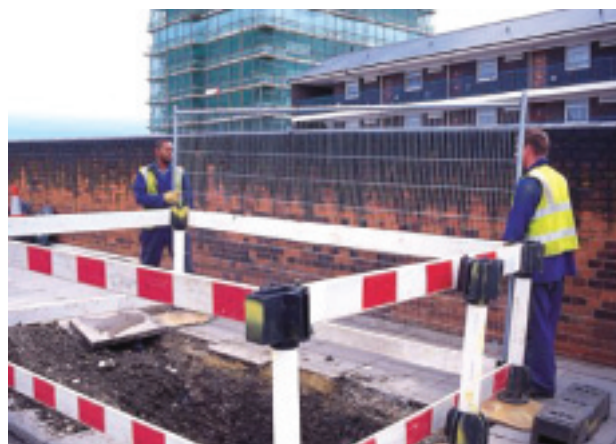
Best Practice in guarding of street works (Source: NJUG)
