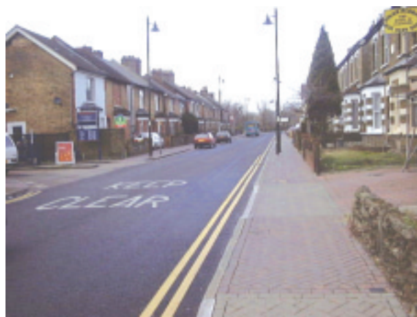
Reinstated footway completed to a high standard (Source: London Borough of Bromley)
