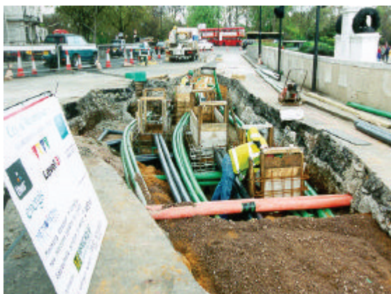
Trench sharing carried out by the telecommunications company THUS
