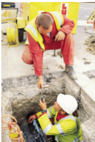
Good quality excavation and tidy work site (Source: NJUG)
