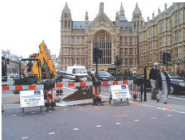
Pedestrians negotiating street works (Source: THUS Telecommunications)
