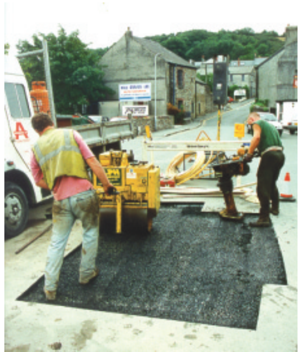
Good compaction technique used on typical asphalt material (Source: TRL Limited)
