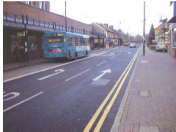
Good quality reconstruction work to the carriageway (Source: London Borough of Bromley)
