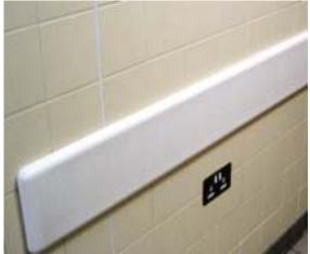
is in use, consideration shall be given to additional horizontal protection at a lower level of approximately 300mm, extending up to 500mm AFFL. The fittings to be sealed at the top and lower edges with the ends stopped to prevent harbourage of pests.
