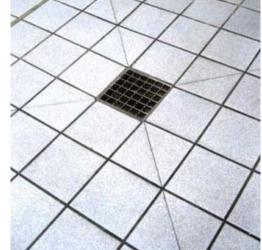
Ponding or pooling of water is not acceptable as stated in food hygiene regulations. Falls away from the floor gully or pools of water at the room perimeters or corners are not acceptable.
