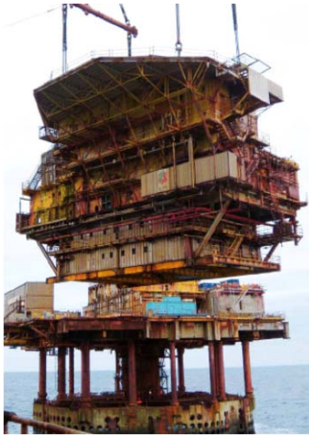
Figure 41. Four modules in one combine lift
