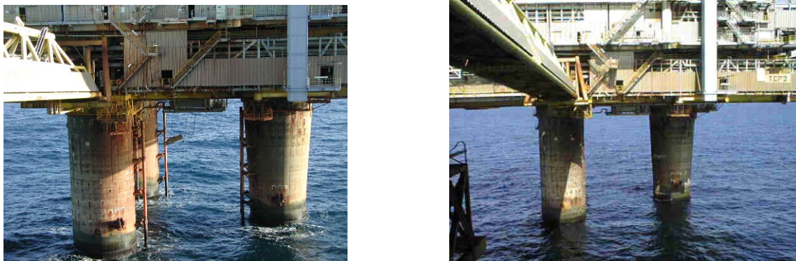
Figure 25. Before and after the removal of utility risers and ladders on one of the TCP2 concrete columns.
