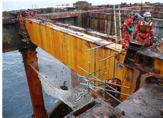
Figure 42. Towards the end of removing the topside facilities
