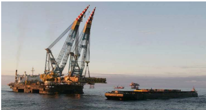
Figure 23. S7000 lifting TCP2 MSF in a single lift
