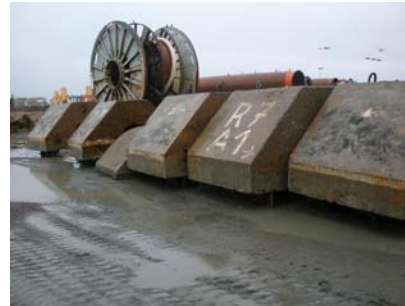
Figure 44. Concrete saddles removed from pipelines
