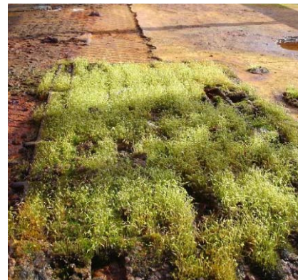
Figure 40. Grass found growing on the steel deck
