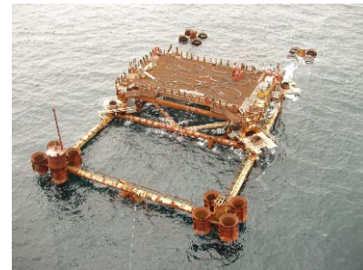
Figure 15. Work platform on DP1 jacket
