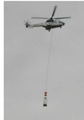
Figure 67. Helicopter testing the installation procedure
