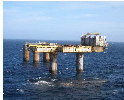
Figure 34. Last module ready for removal by S7000
