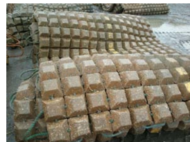
Figure 27. Concrete mattresses removed
