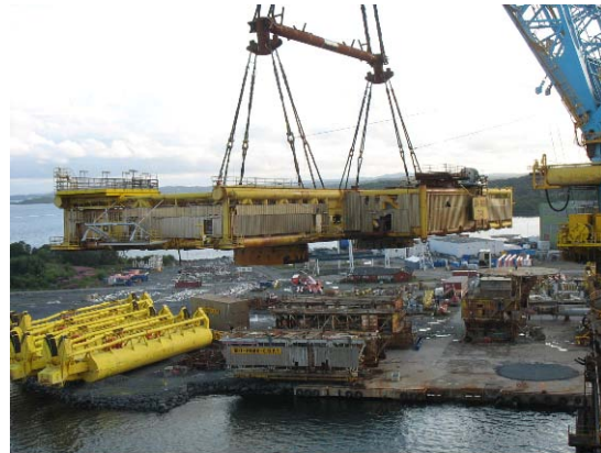
Figure 36. TP1 MSF loaded onto the Aker Stord disposal Yard by S7000
