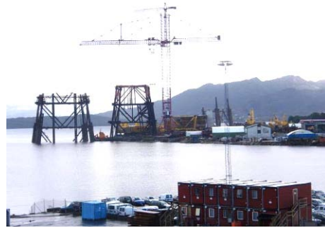
Figure 31. QP Jacket at the disposal yard
