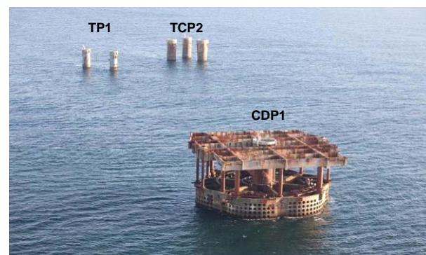
Figure 3. Frigg Field after offshore removal works
