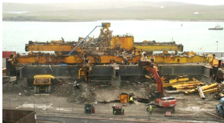
Figure 46. TCP2 MSF at the onshore disposal facilities at Lerwick, Shetland
