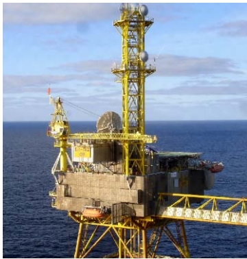
Figure 28. QP Topside before removal
