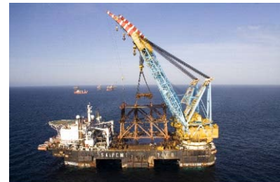
Figure 16. Upper part of DP1 jacket lifted off by S7000
