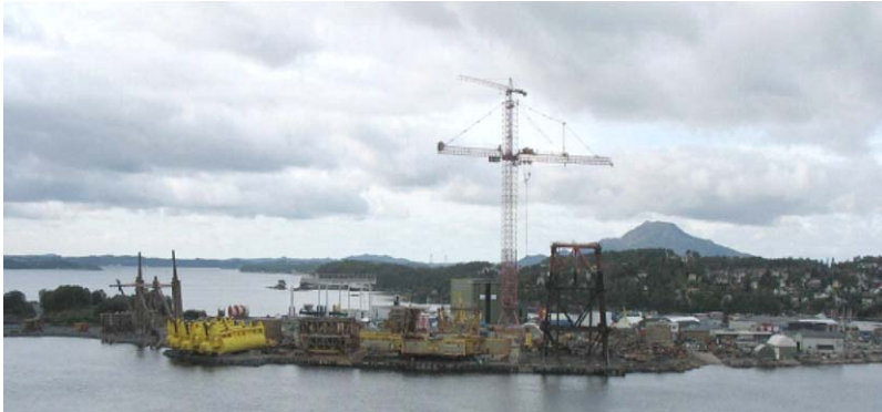
Figure 45. Onshore disposal facilities at Aker Stord, Norway
