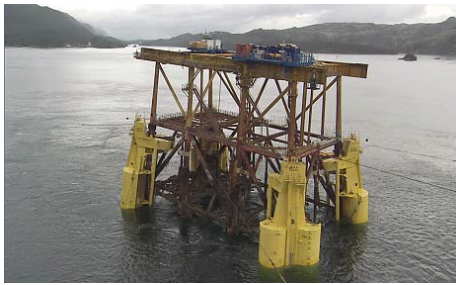
Figure 11. DP2 Jacket and MSF tow arriving the inshore location
