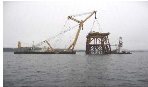
Figure 12. DP2 MSF being lifted off
