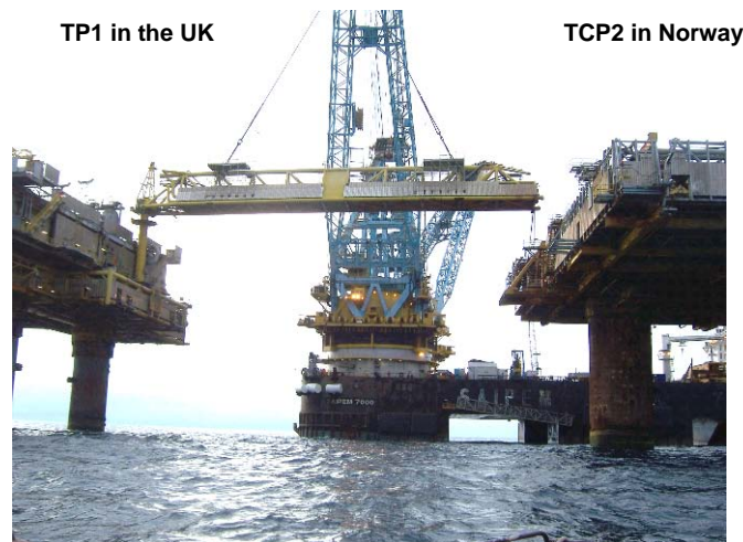
Figure 1. Removing the bridge crossing the border between the UK and Norway on Frigg
