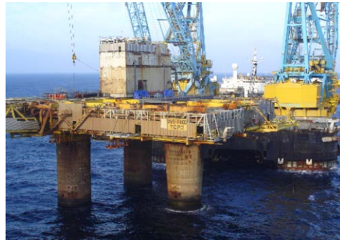
Figure 20. Last module being lifted off TCP2 MSF
