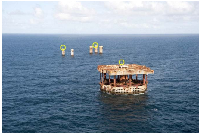
Figure 68. AtoN configuration on Frigg concrete substructures, the positions of the AtoN are shown in yellow circles
