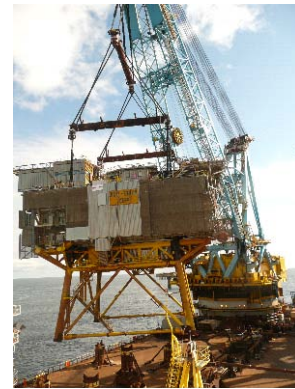
Figure 29. QP Topside and MSF being lifted onto the deck of S7000
