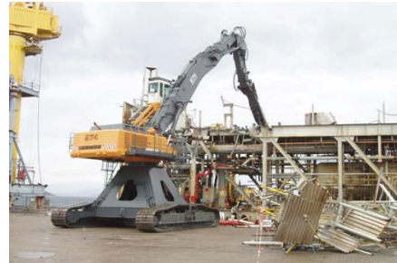
Figure 49. Demolition of modules using large excavators
