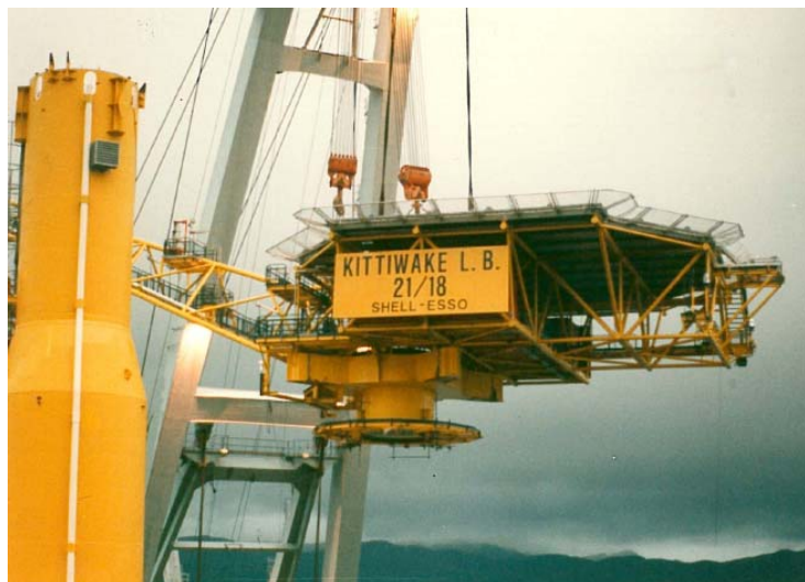
Figure 7.12 Kishorn 1990 Installation of Rotating Head
