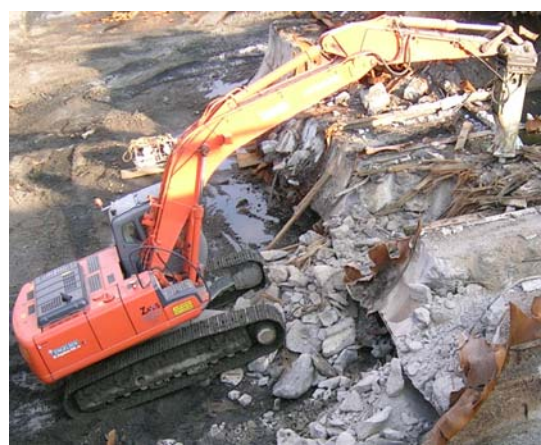
Fig 7.14 Breaking Concrete Ballast
