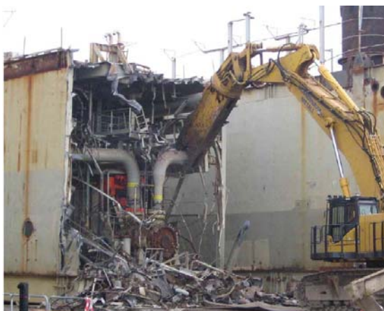
Fig 7.13 Cutting with Hydraulic Shear
