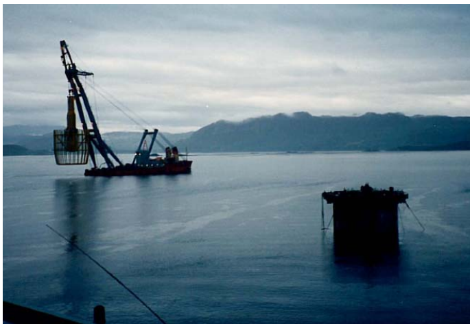
Figure 7.11 Kishorn 1990 Installation of Pedestal & Fender
