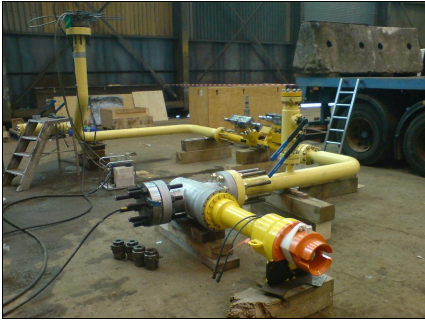
Figure 17: Photograph of the flowmeter spool piece.
