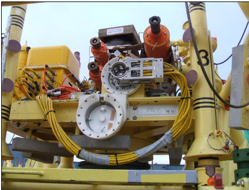
Figure 13: Onshore mock-up of the Tristan NW umbilical control panel and jumpers.
