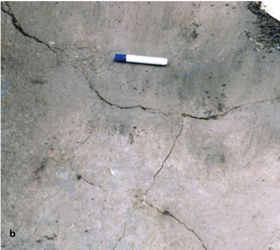
(b) Map pattern cracks in sulfate-attacked oversite concrete beneath a suspended wooden floor of an adjacent room.
