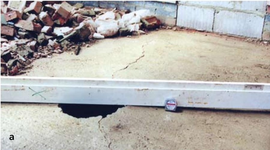
**Figures 7(a, b & c):** Sulfate-attacked oversite concrete that was laid over plaster contaminated brick rubble beneath a suspended wooden floor (here removed together with the sleeper walls).
