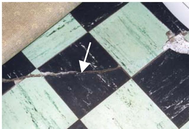
**Figure 9:** Stepped crack in floor of 1950s house that may indicate sulfate attack. The unevenness could be felt through the (rolled back) carpet.
