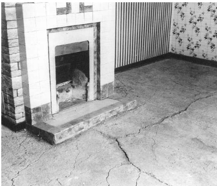
**Figure 1:** Distortion and cracking of a concrete floor slab caused by sulfate attack. Damage is greatest in front of the fireplace where water, carrying sulfates from underlying hardcore, has been drawn through the slab by heat from the fire.
