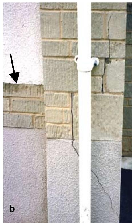
**Figures 8(a & b):** Exterior of a bungalow affected by sulfate attack in South Wales. The worst damage is on the downslope side where there is about 1 m of exposed masonry below internal floor level.
