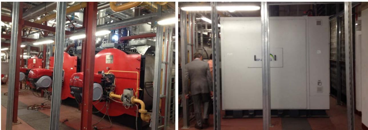
**Figure 3: The Homerton CHP installation (right), and the new boilers (left)**
