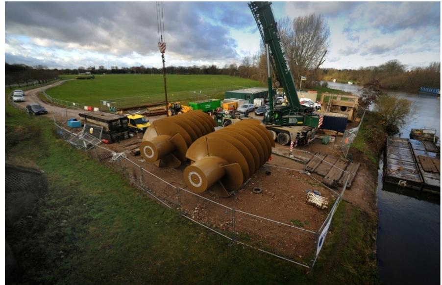
Two 40-tonne Hydropower turbines installed at the Environment Agency's Romney Weir on the River Thames.
