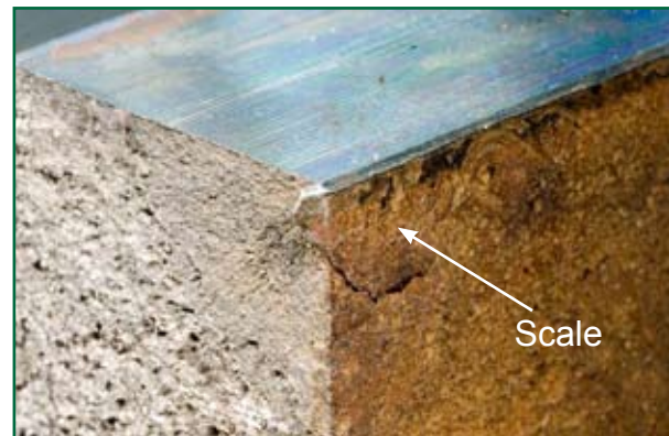
Figure 8: Detail of fracture origin and adjacent 'scale' at edge.
