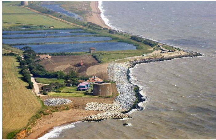
Figure 1.3 Completed East Lane, Bawdsey Coast Protection and Flood Defence Scheme (source: M Page)
