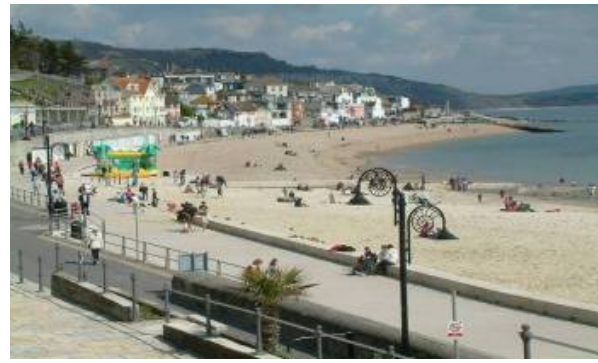
Figure 1.5 Completed seawall, beach and jetties (image courtesy of Environment Agency)
