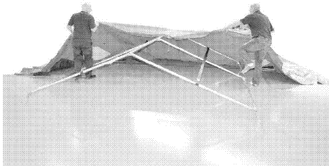
Fig 18 Place canvas over roof frame (typical arrangement)
