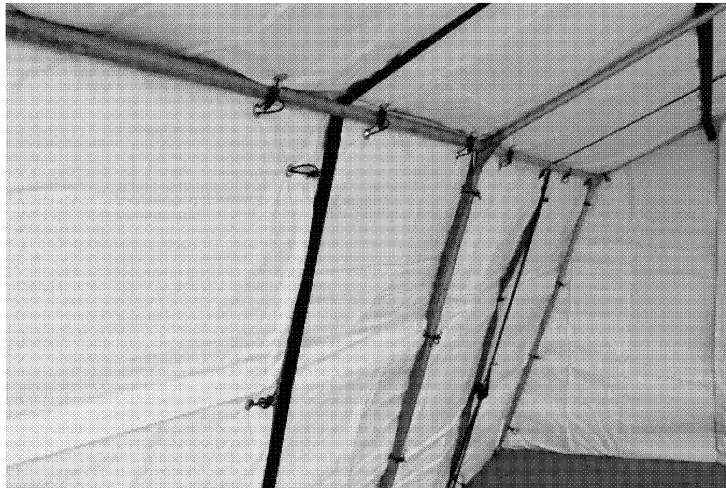
Fig 24 Wall insulation panel (Typical arrangement)
