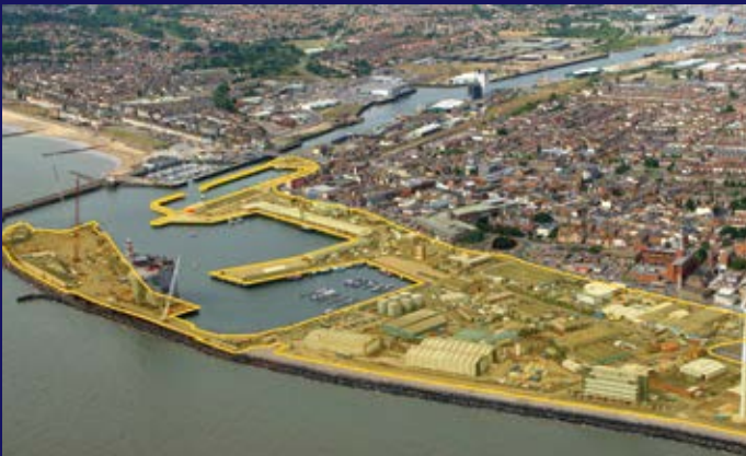
Lowestoft Power Park
