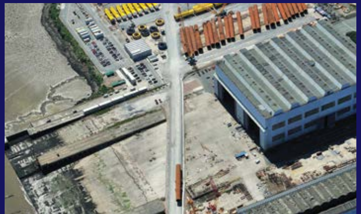
Cammell Laird Ship Yard
