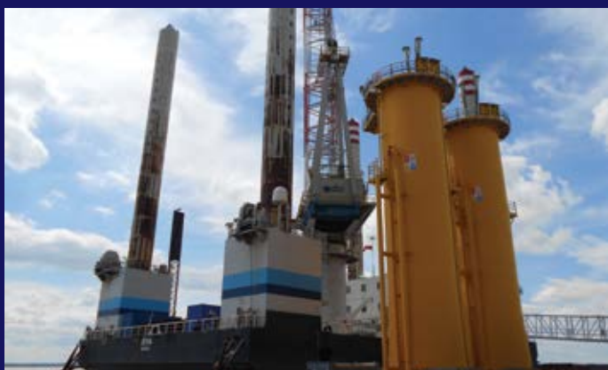
Load out of transition piece at Port of Grimsby
