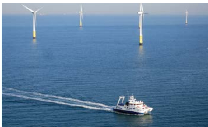
Survey work being undertaken by Osiris Projects using Bibby Tethra
