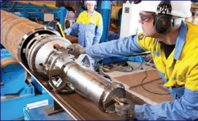
TATA Steel has a new £2m offshore processing centre (OPC) producing welded tubular assemblies for jacket foundations.
