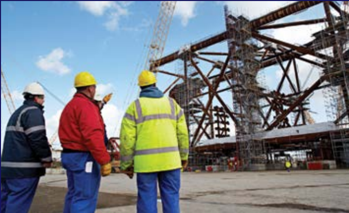
Jacket construction at OGN, Wallsend
