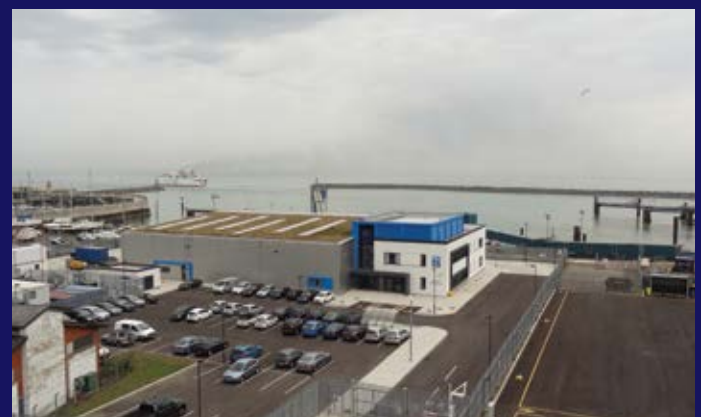
London Array O&M base at Port of Ramsgate
