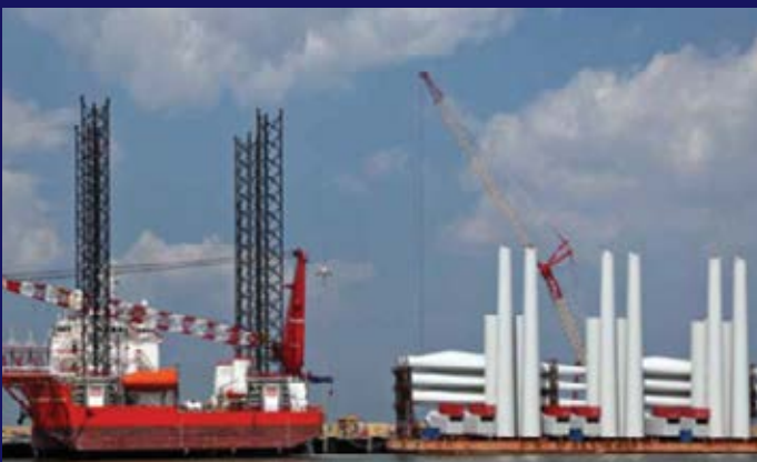
Blades and Towers Great Yarmouth
