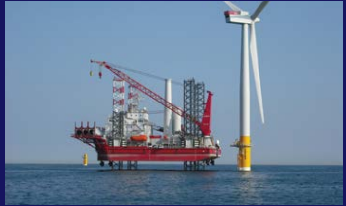
Seajacks installing Greater Gabbard
