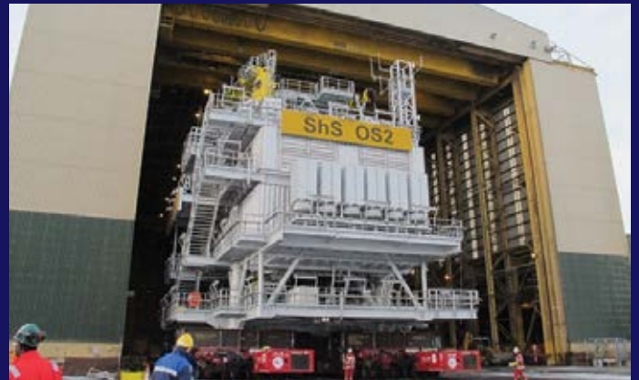
Substation loadout at Heerema Fabrication Yard, Hartlepool
