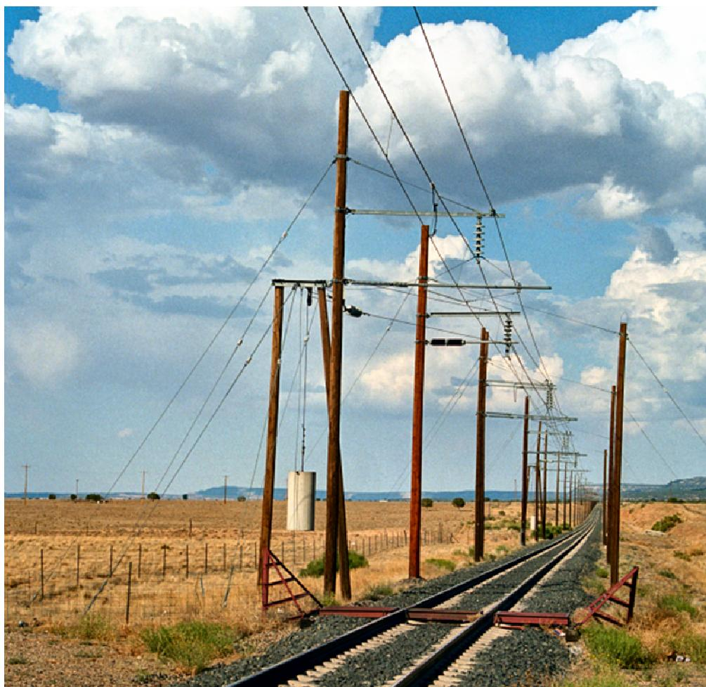
**Figure 3 Wooden Poles Supporting Catenary on the BM&LP Railway**
