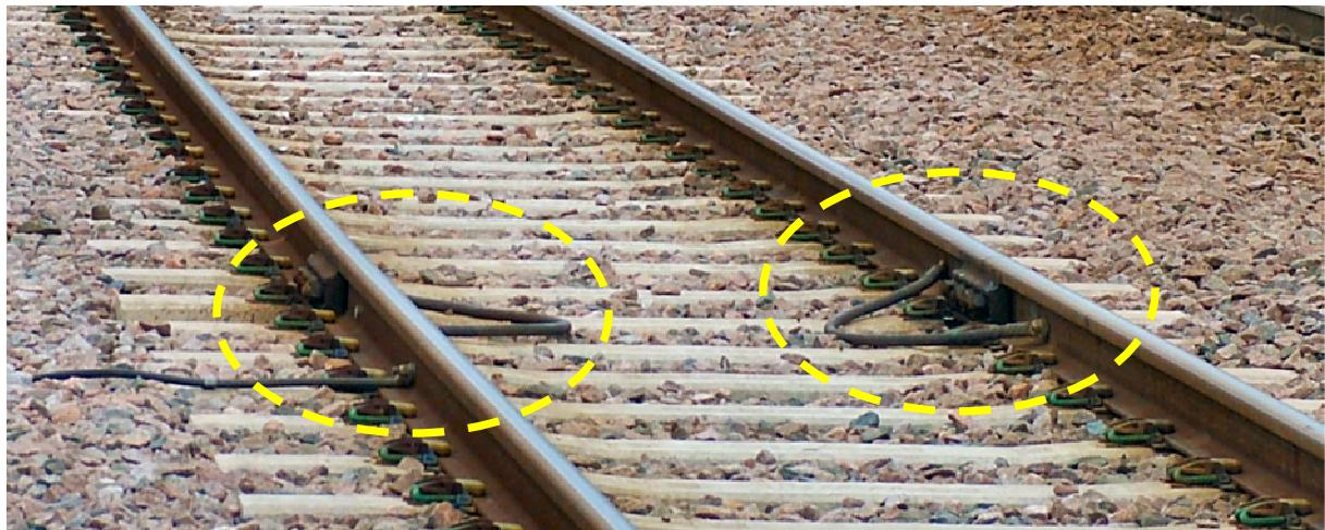
**Figure 15 Jumpers Across Fishplated Rail Joints**
