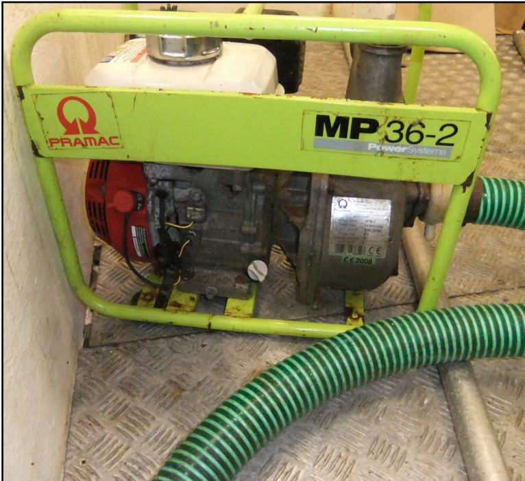
Figure 1: The petrol engine-driven salvage pump
