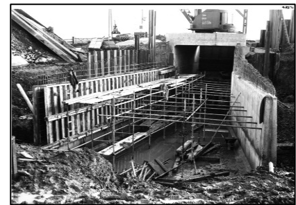
Monk's Leaze Clyce inlet sluice under construction
