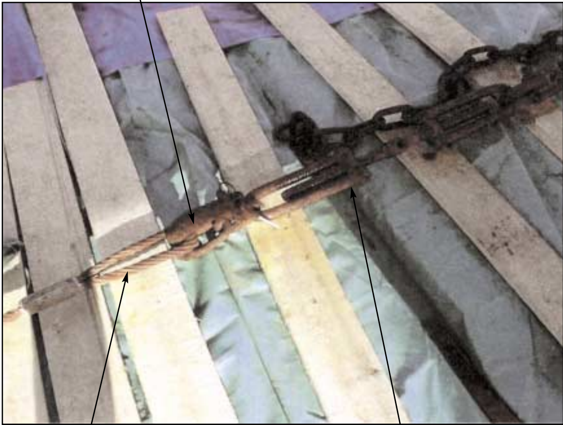
End loop in wire lashing
