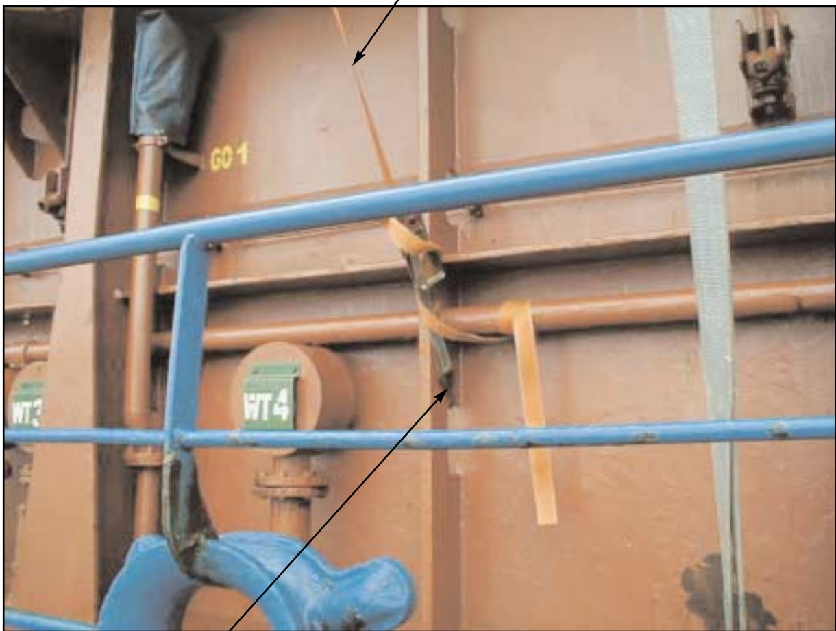
Not a proper securing point
