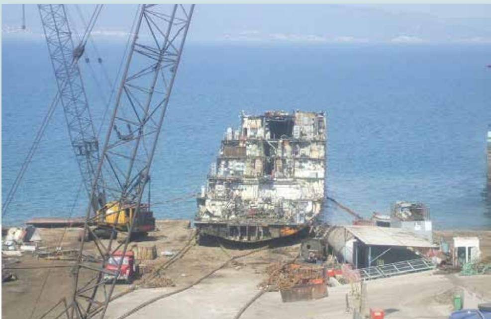
25/03/2014 Cumberland was the last vessel to be recycled shown here on the slipway, Radar & Superstructure now removed.
