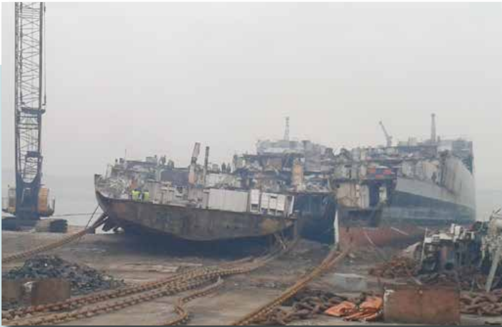
28/01/2014 Chatham in the foreground in the final stages of dismantling
