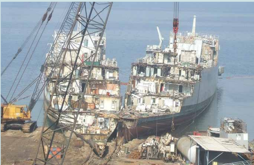
17/02/2014 From left to right Cumberland & Campbeltown on the Slipway.
