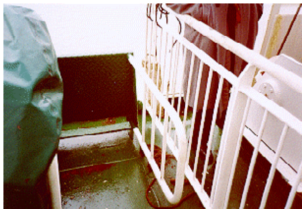
Boarding Bridge in "Closed" Position
