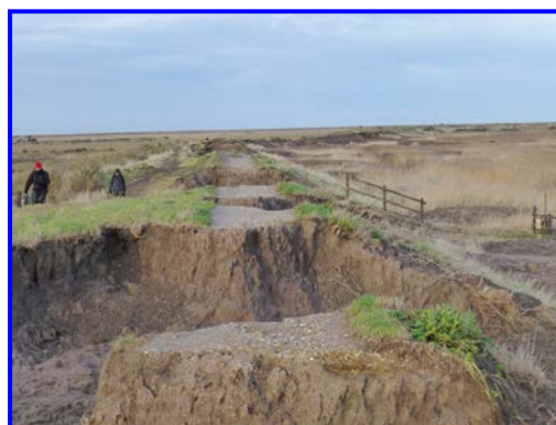
One of the 20 plus breaches in the flood embankment protecting the Blakeney Freshes European Site
