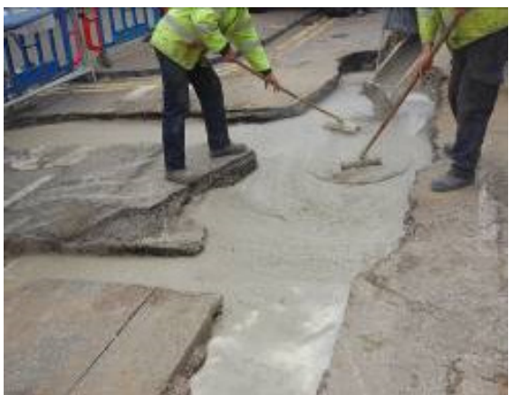
Figure 2 - Foamed Concrete for Reinstatement in use
