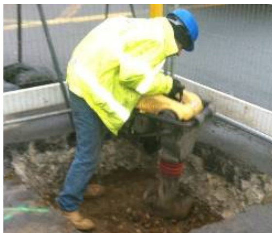
Figure 3 - CBGM being compacted
