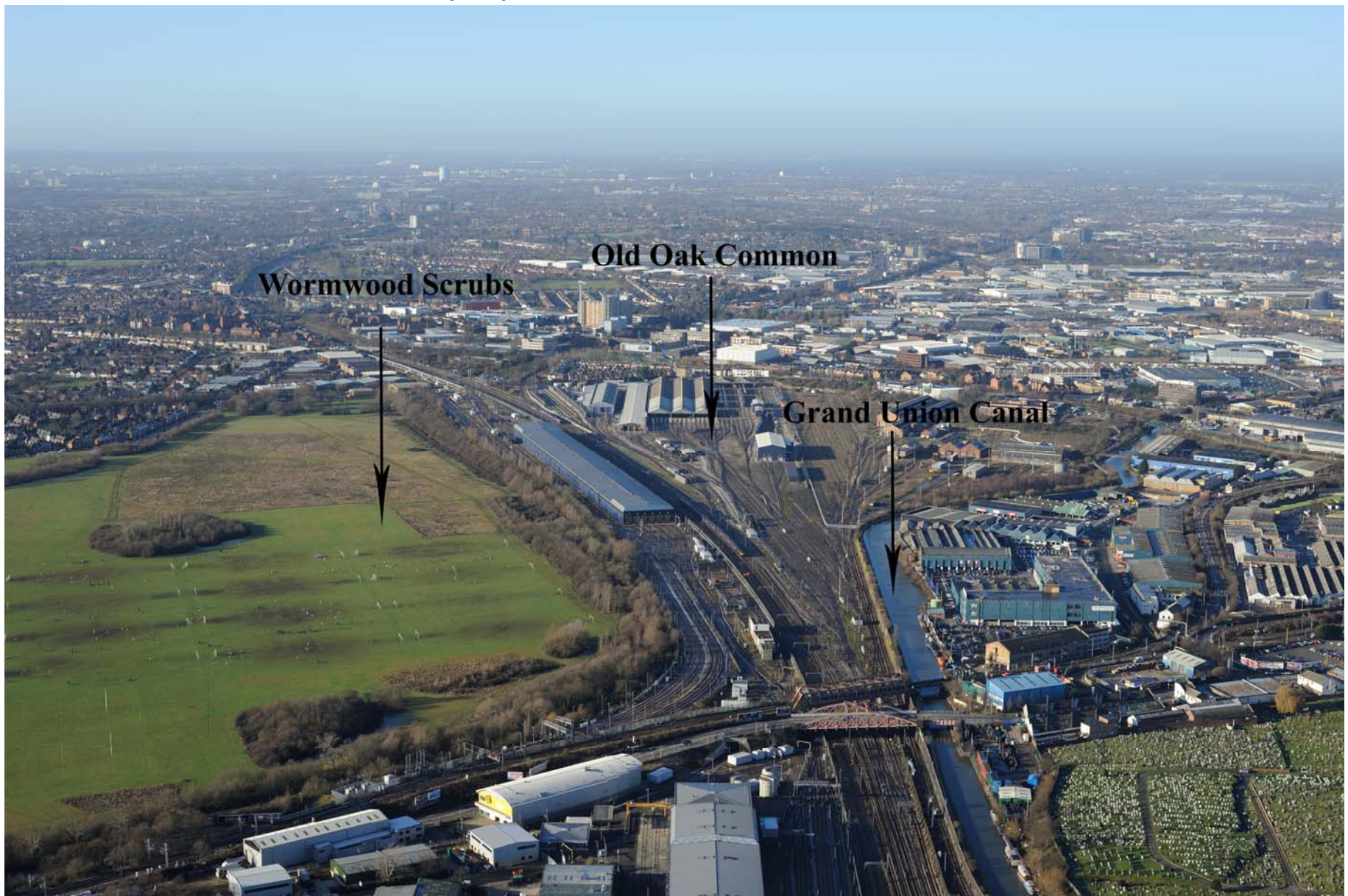
Figure 14 – Aerial view of Old Oak Common [HS2 Ltd]
