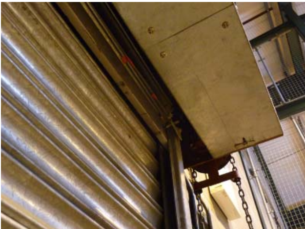
Looking up at top of door showing drop-weight bar in guide rails
