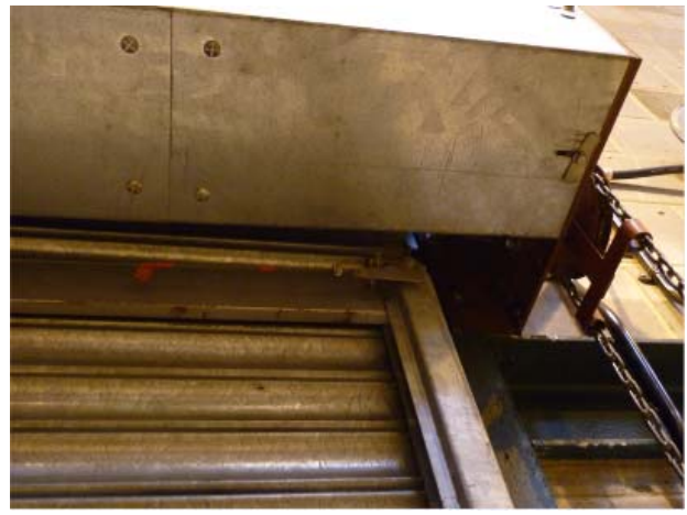
Looking up at top of door showing drop-weight bar support bracket
