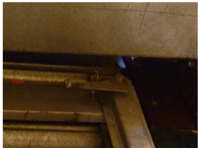
Close-up of bracket supporting steel pin
