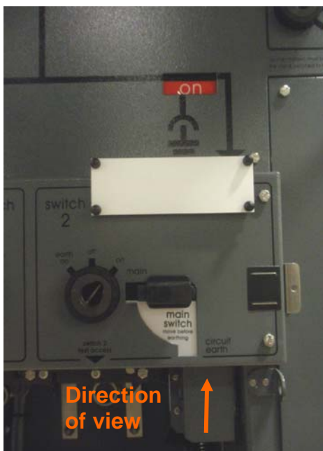
4.8 RSW2 Service position Main selected Main ON
