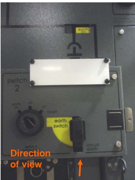
4.20 RSW1 Service position Earth selected Earth ON
