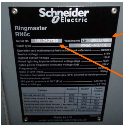
Data plate on the LV cabinet of the Ringmaster
