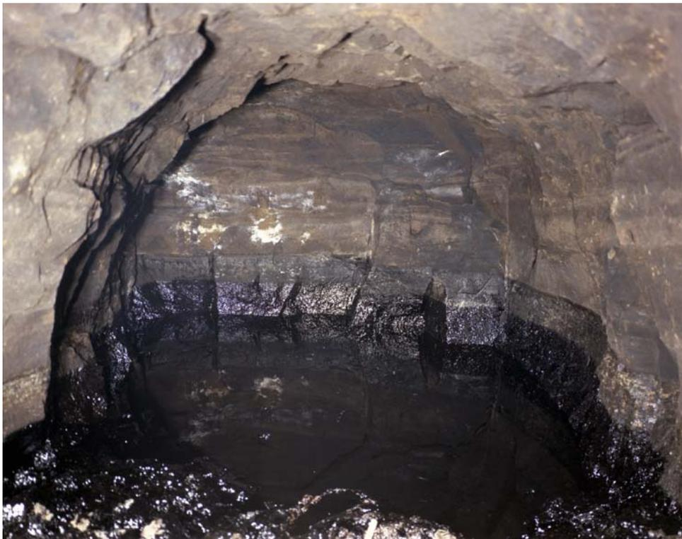
Figure 4.1 Coalport Tar Tunnel- one of the collection pits of a small, mined field in the Carboniferous Halesowen reservoir, exploited in the 18<sup>th</sup> century. The tunnel was opened up to bring out coal from below ground to the Severn River in Coalbrookdale, Shropshire (© NERC).
