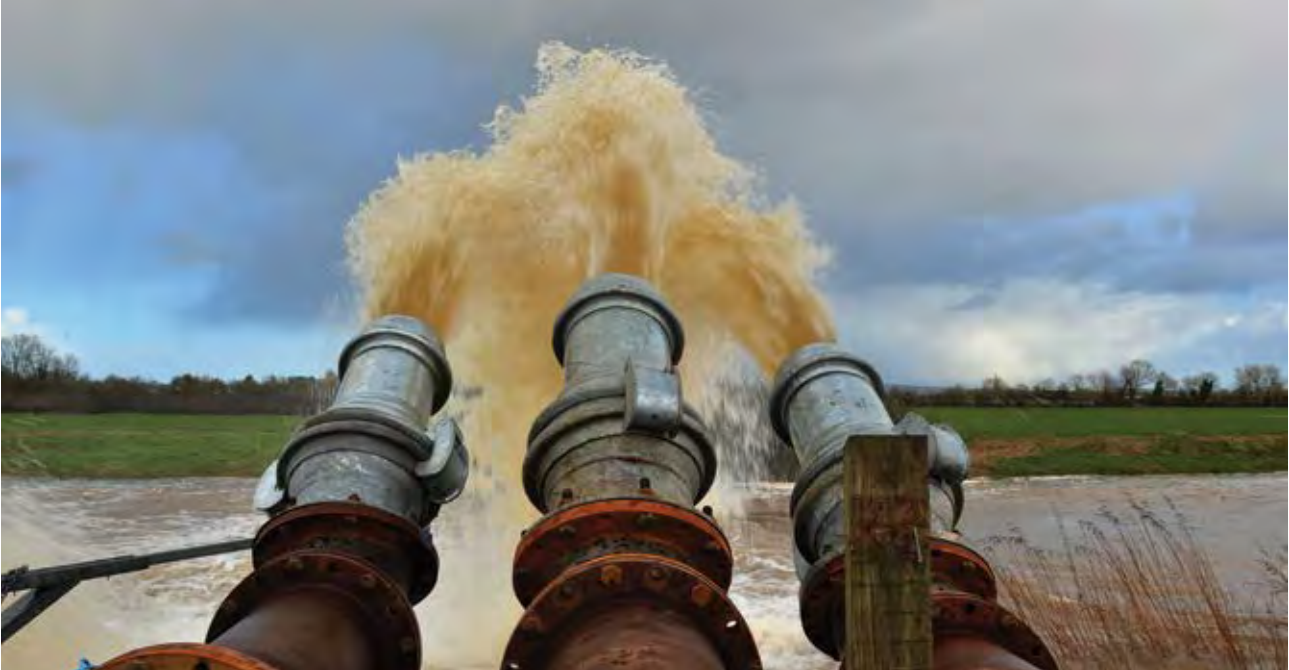
Floodwater is pumped into the River Parrett at the Saltmoor Pumping Station near Burrowbridge in Somerset © Crown
