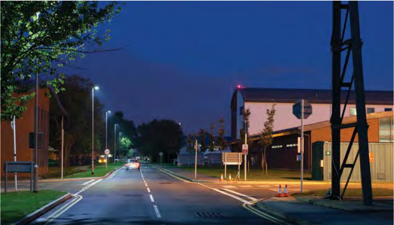
RAF Northolt, one of fifteen sites to have shared a £1.7m investment in external LED street lighting © Phillips
