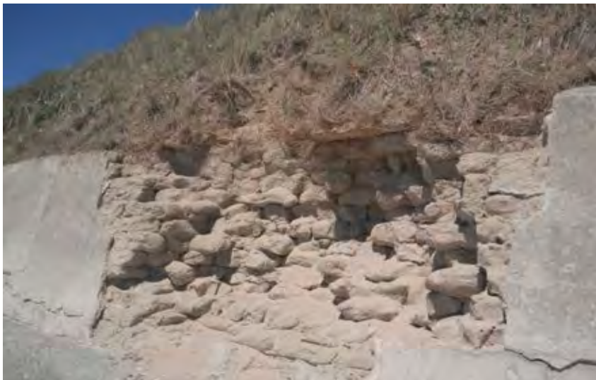
Damaged sea wall Cymyran Beach RAF Valley © Crown
