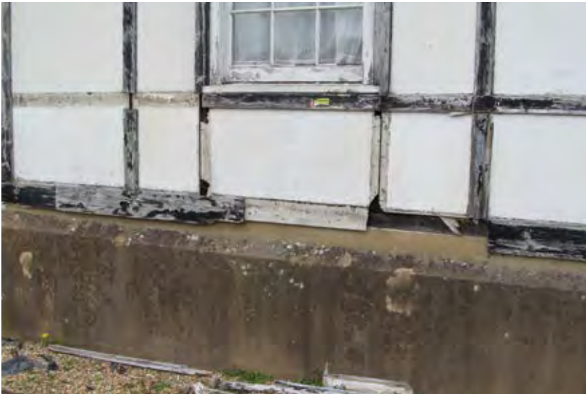
Typical defects © Aspire Defence Services Limited
