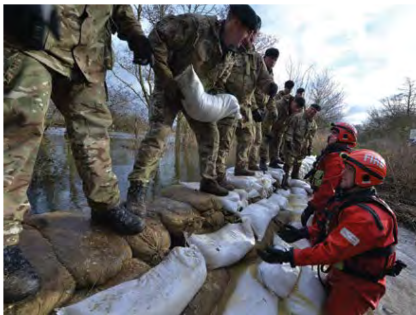
Reserve Soldiers of the 7th Battalion The Rifles assist Berkshire Fire Brigade to dam a breach in the Kennet Canal that threatened an electrical sub-station near Burghfield, south of Reading during flooding in February 2014 © Crown
