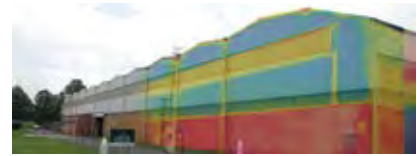
Warehouse thermal imagery © Crown
