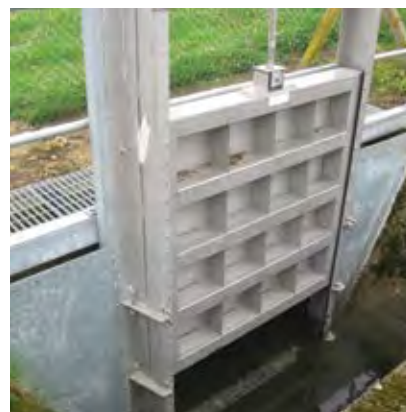
Penstock Valve protecting the River Yeo against spillages © Crown
