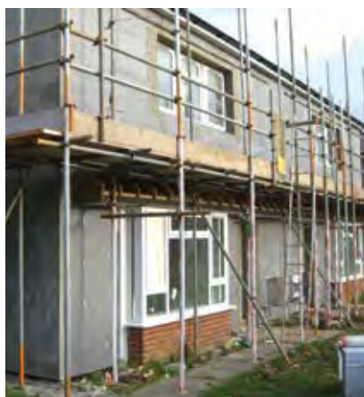
Refurbished Service Family Accommodation at Bulford © Crown
