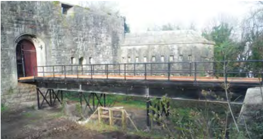
The new replacement bridge 2013 © Crown
