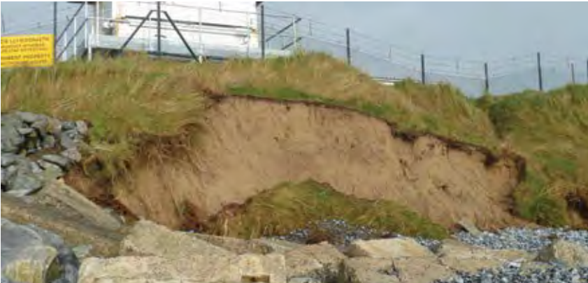
Dune erosion caused by tidal surges © QinetiQ
