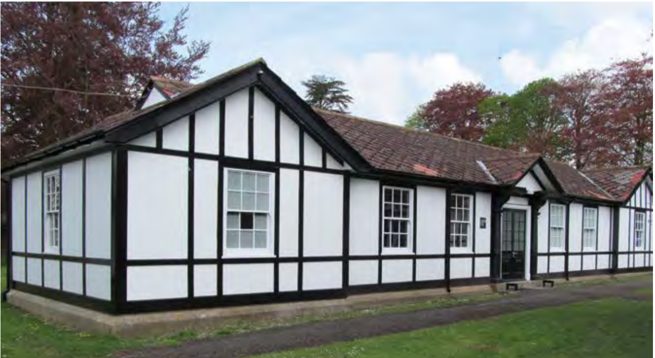
Work is complete © Aspire Defence Services Limited
