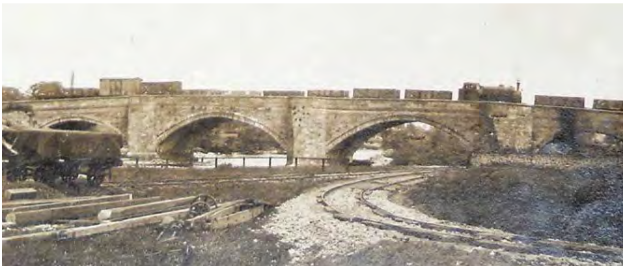
A train travelling on the medieval road bridge over the River Swale at Catterick. The road bridge was constructed in 1421 during the reign of Henry V. Five hundred and one years later, in 1922, a purpose-built railway bridge was constructed (Courtesy of Henry Boot Plc)
