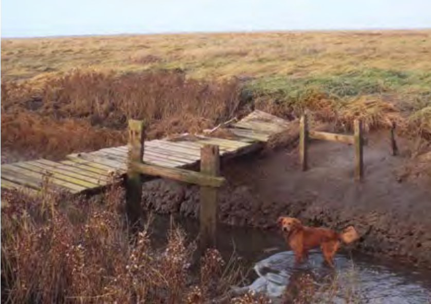
Damaged bridge caused by tidal surge © Graham Wall
