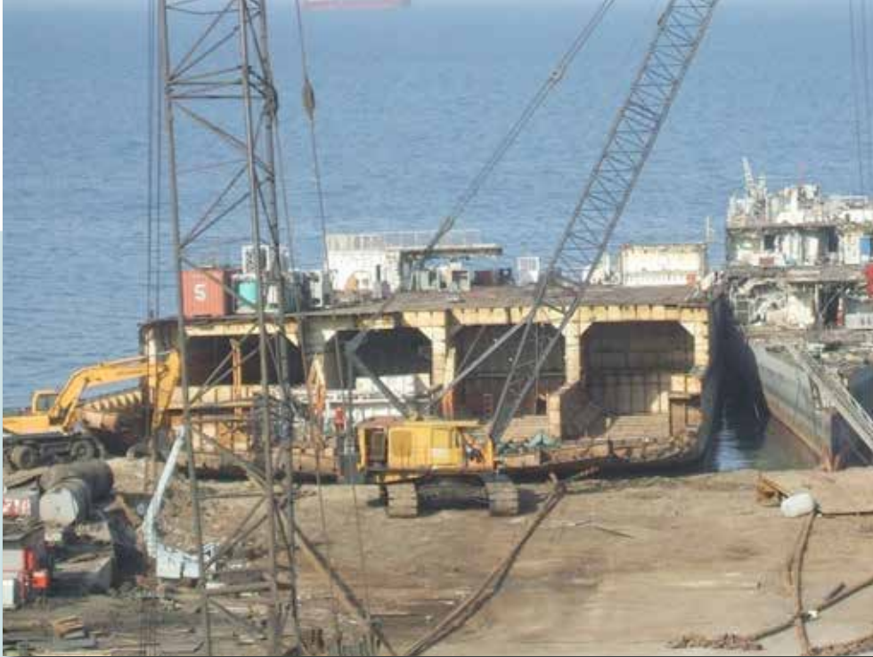
Longbow progress of works 26/12/2013
