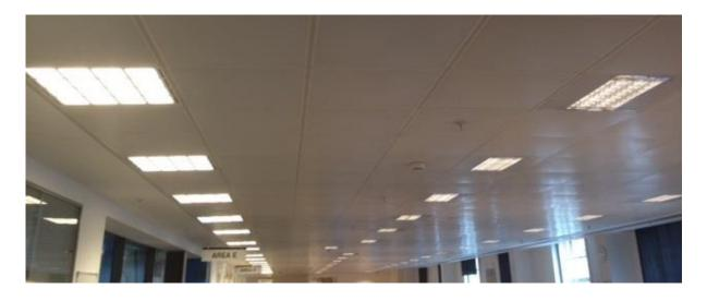
The new LED lighting is shown (on the left hand side) alongside the old T5 fluorescent fittings in the photo above taken during the course of the refit.
