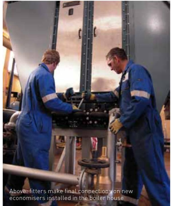
Above: fitters make final connections on new economisers installed in the boiler house
