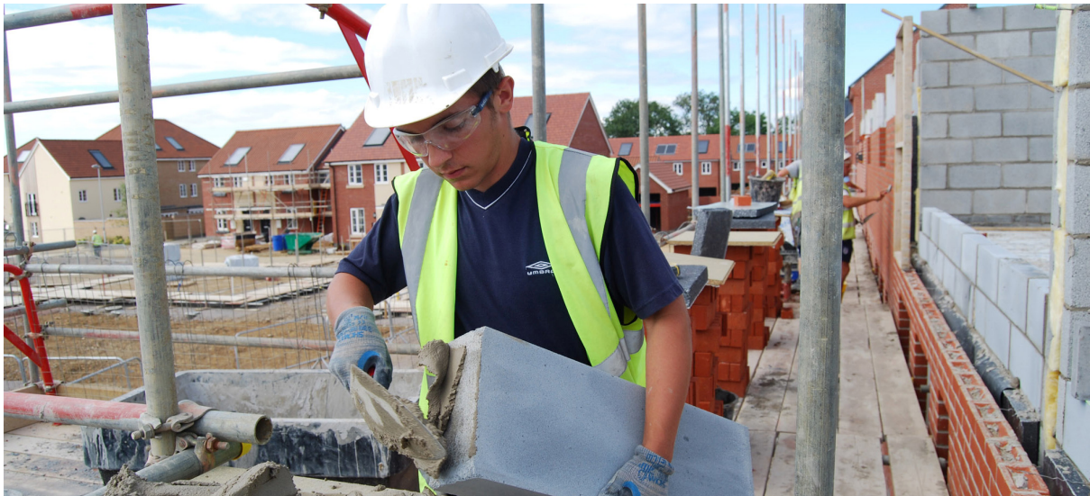
David Tompkins, Construction Futures trainee
