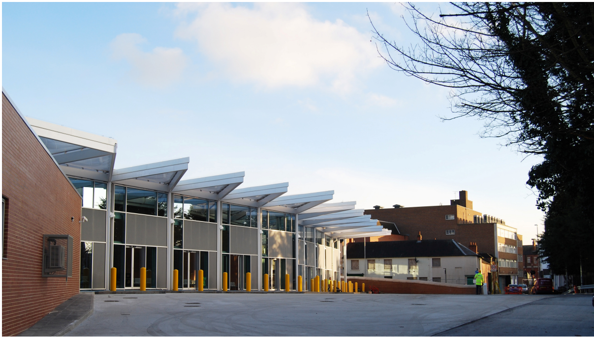
North Gate Bus Station, close to completion
