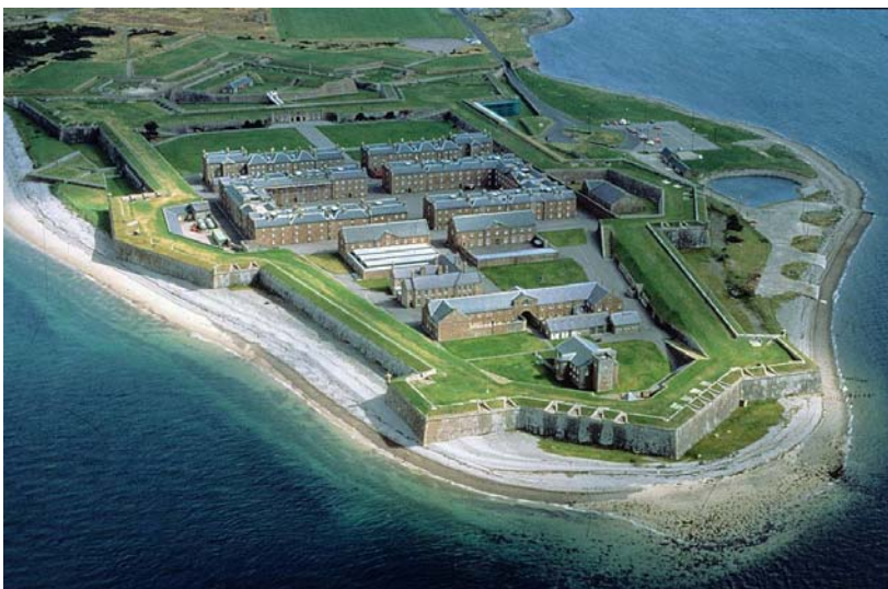
Figure 2 Fort George barracks in the image, are at risk of coastal erosion
