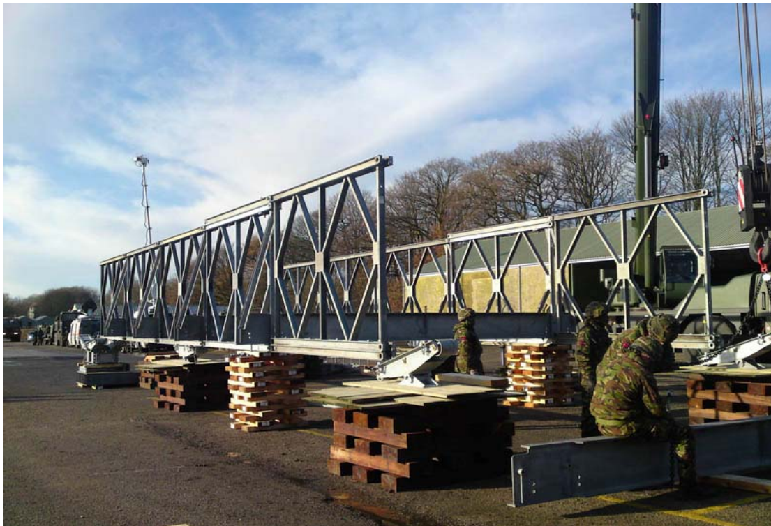
Figure 2 Soldiers from 3 Armoured Engineer Squadron work on the temporary footbridge to span the River Derwent (Cumbria) after severe floods in Nov 09 damaged various bridges across the area leaving communities with no easy access to essential services. The UK CCRA has identified that there would be added burdens on UK emergency services in responding to more frequent flooding, heatwaves and wildfires (Picture: Kevin Hegarty, Crown Copyright/MOD 2009).
