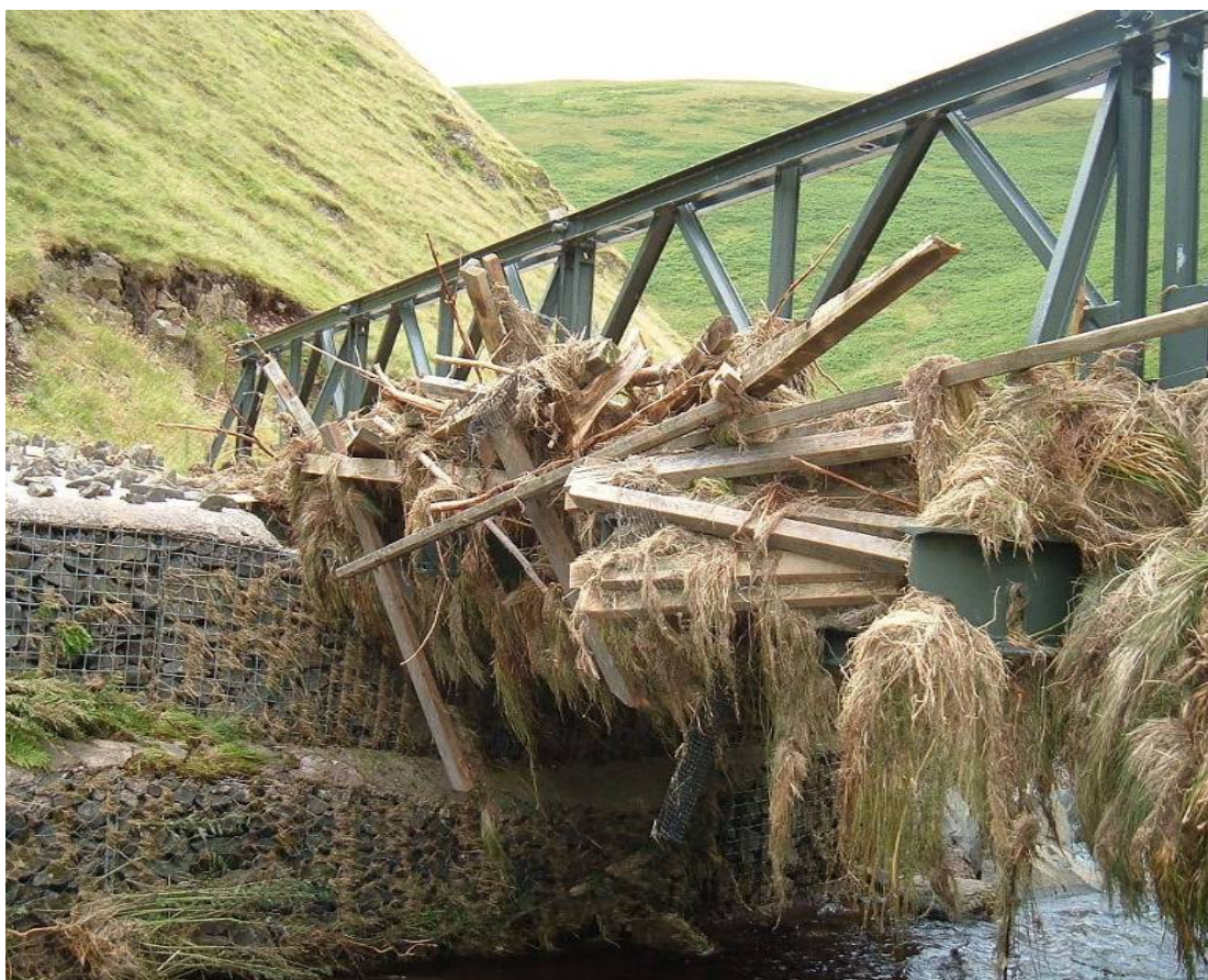
Figure 7 Bridge (in the photo), track and riverside damage by flash flooding at DTE Otterburn caused training disruptions and increased relief costs
