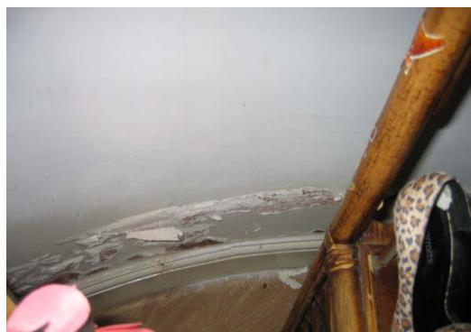
**Top left:** condensation and mould growth, caused by a mixture of inadequate heating and lack of room ventilation
