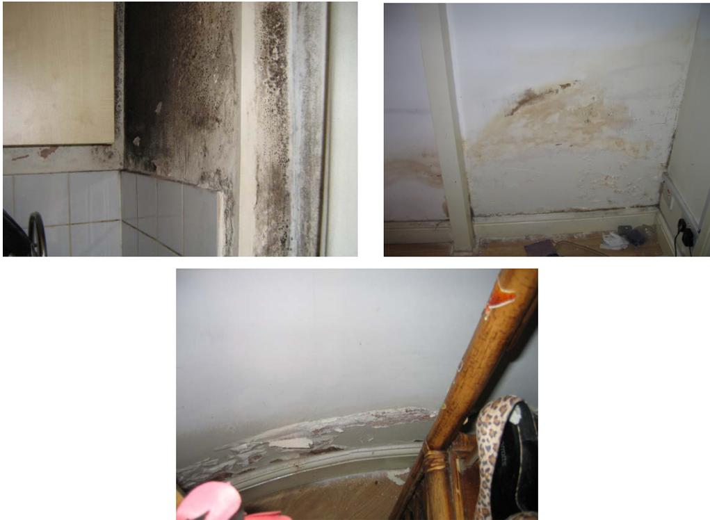
**Top left: condensation and mould growth, caused by a mixture of inadequate heating and lack of room ventilation**
