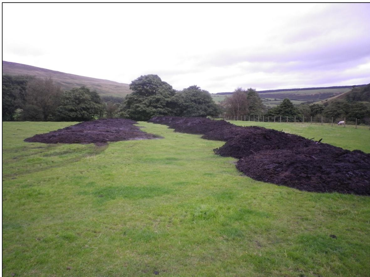
**Plate 7.1: Example of shorter term stockpiling of dredged material prior to spreading** (note this photograph is not based on the Somerset Levels area and is intended to represent
