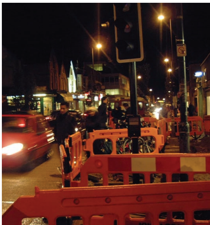
Figure 8.2 Night-time removal of traffic management in Oxford (Oxfordshire CC)
