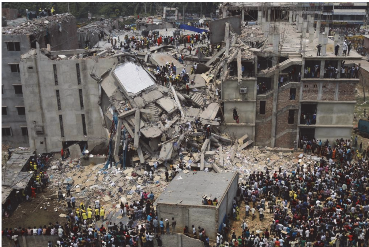
Dhaka: collapse of Savar building (Rana Plaza). Photo credit: Jaber Al Nahian.
