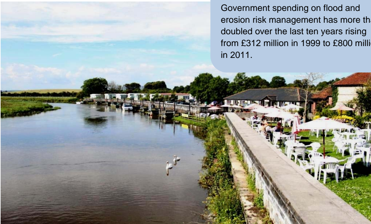
The River Arun, upstream of Houghton Bridge
