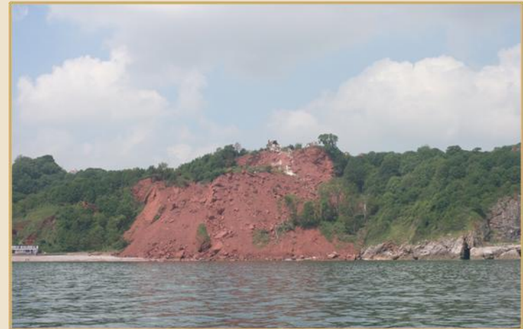
Recent landslide at Oddicombe Bay
